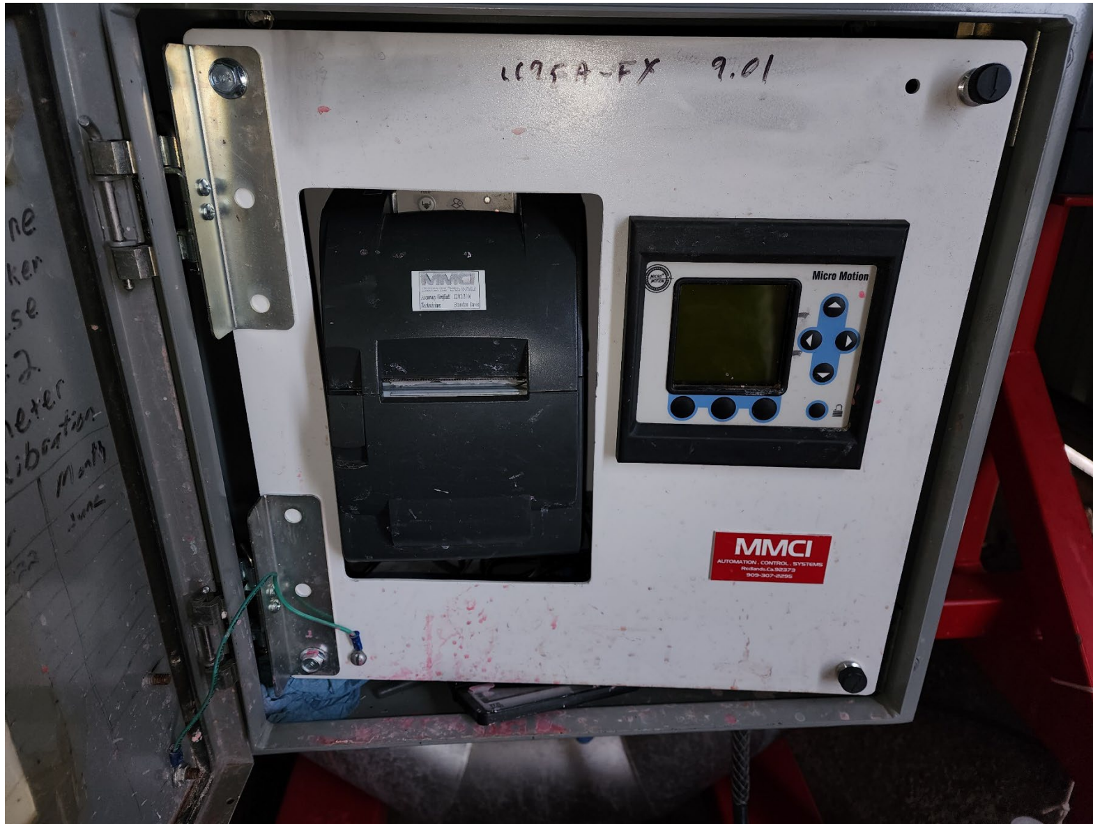
MicroMotion meter setup inside control box
